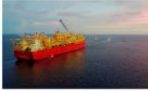
Shell Prelude FLNG Australia
